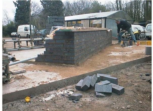
A variety of panels were built, and a range of materials used. Above we have one of the corner panels in engineering brickwork.
